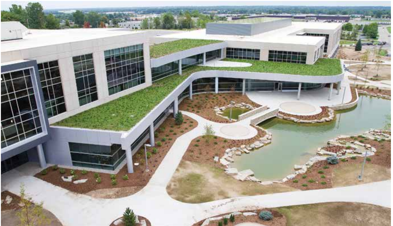
The 384,000-square-foot facility features two rectilinear wings, two and three stories tall, that meet at an angle at a central three-story lobby. The 50,000-square-foot 'Connector' atrium includes a rooftop plantings. Photo: Craig Van Wieren.
